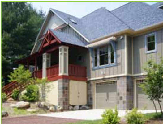
First home in Pennsylvania to be LEED certified. LEED is an internationally recognized green building certification system.
