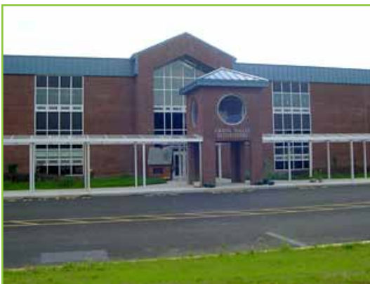
Green Valley Elementary School. SMCA contractor performed testing, adjusting and balancing of all air and hydronic systems.
